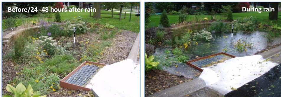
Figure 4: Rain garden before/after and during a rainfall event
