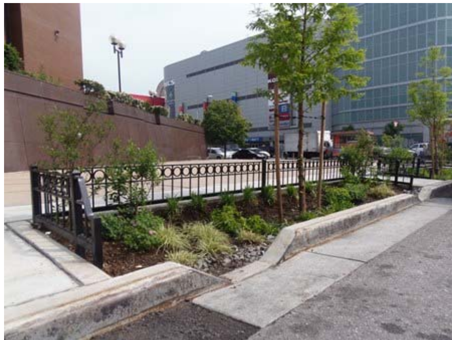
Figure 4: Right-of-way bioswale installed in New York City (NYC Environmental Protection, 2013)
