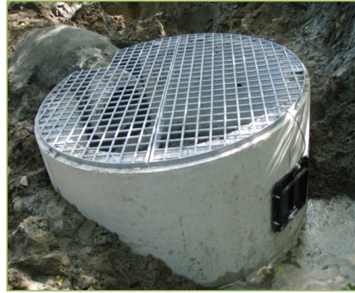
Figure 18: Outlet Control Retrofit
