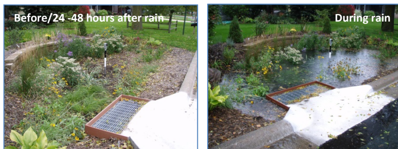
Figure 7: Curb Cut Rain Garden Example
