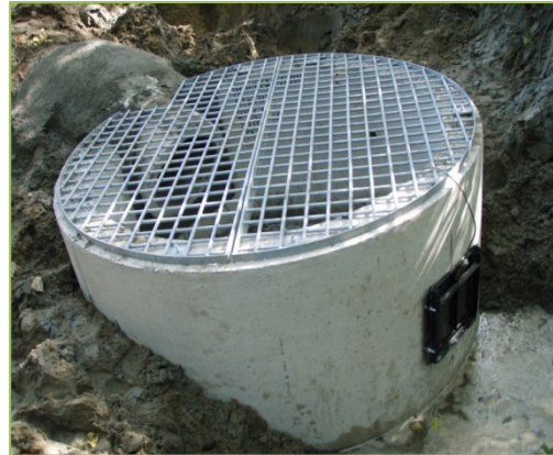
Figure 17: Outlet Control Retrofit
