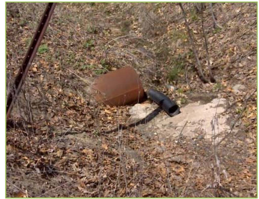
Figure 13: Drain Tile Outlet from Ag. Field
