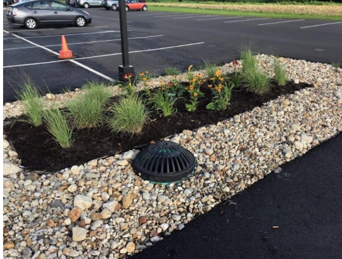
Figure 10: An HPMBs basin installed at a parking lot catch basin. The total footprint of the practice is about the size of one parking space.
