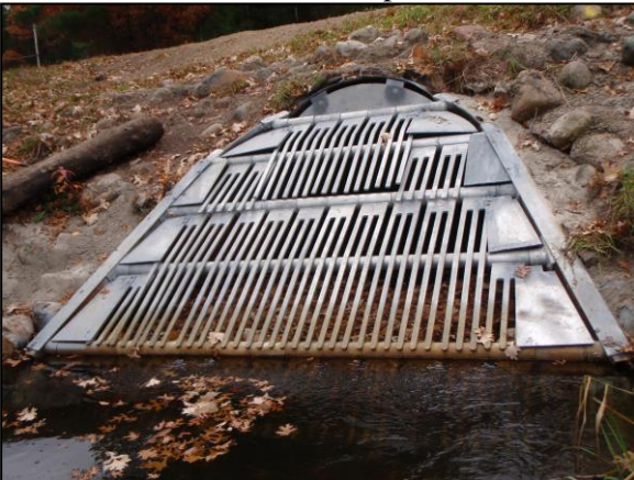
Martin Lake south inlet (completed 2014)
