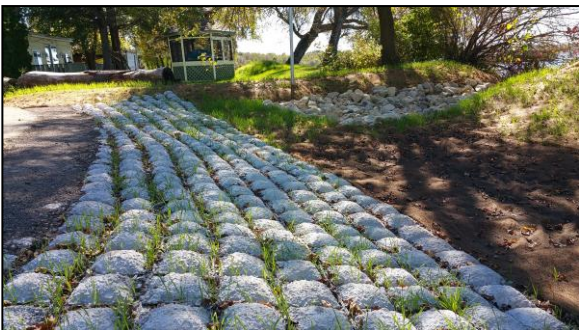
Lincoln Avenue stormwater stabilization.
