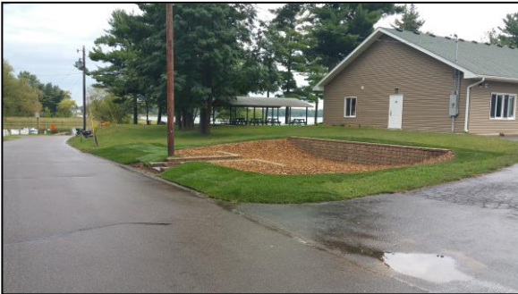
Coon Lake Beach Community Center rain garden
